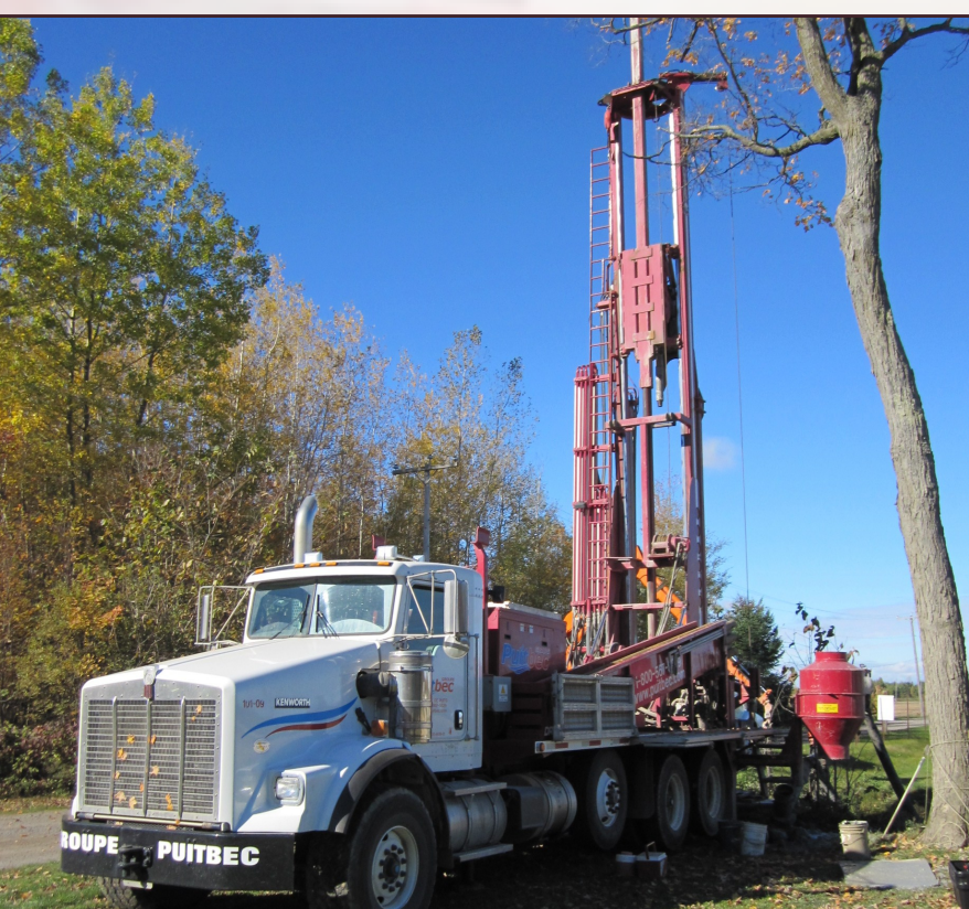
Figure 2: Foreuse Foremost DR-12
