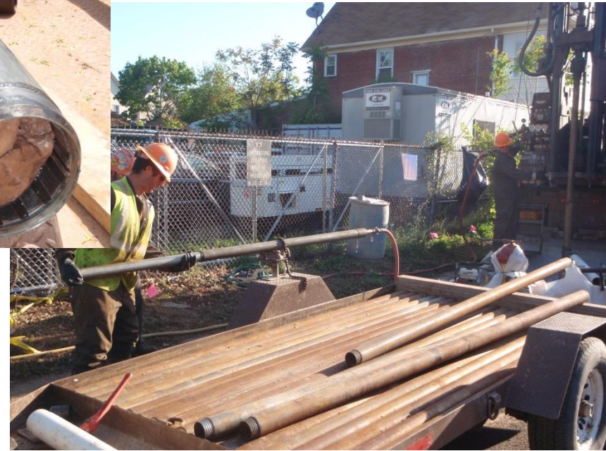
Triple-tube core barrel
